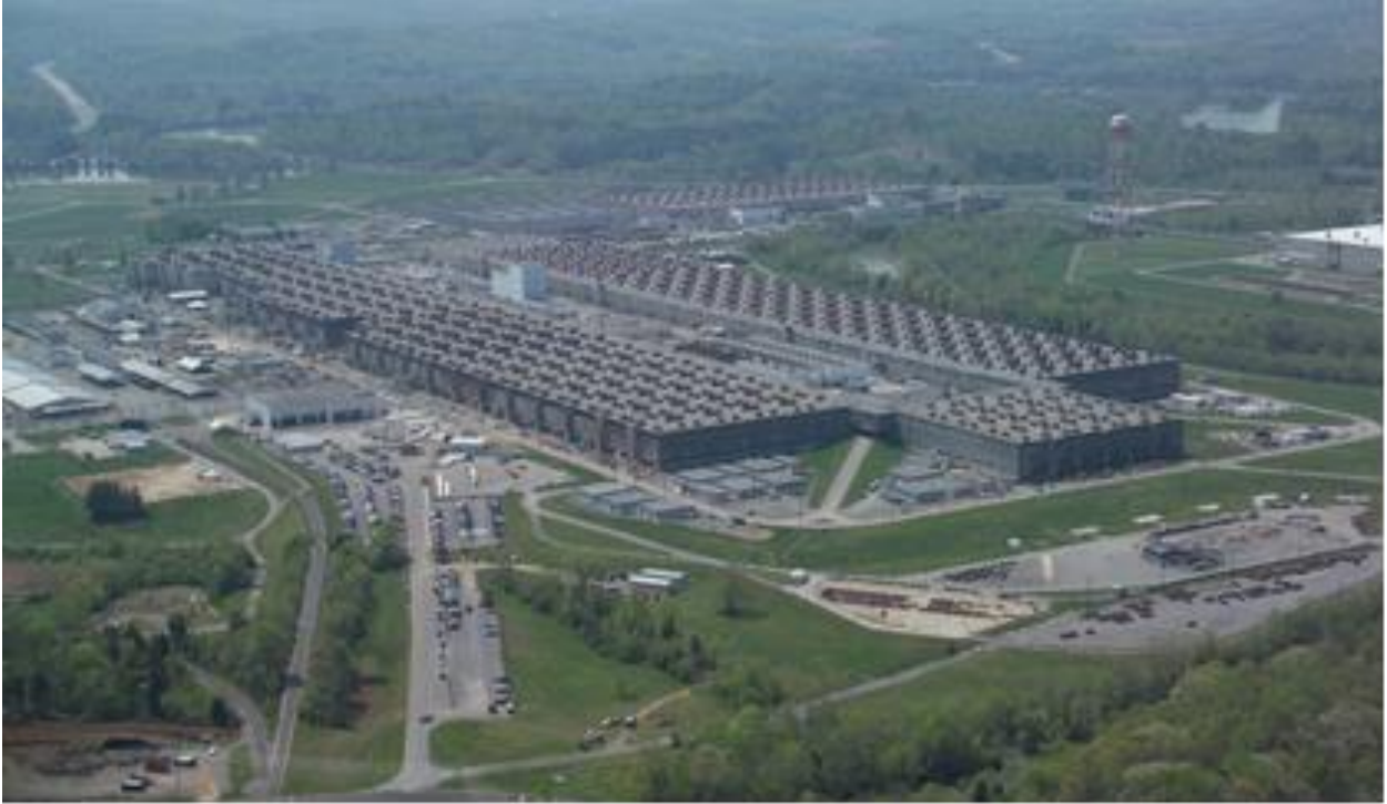
Figure 2. Building K 25, looking southwest, circa 2005.
