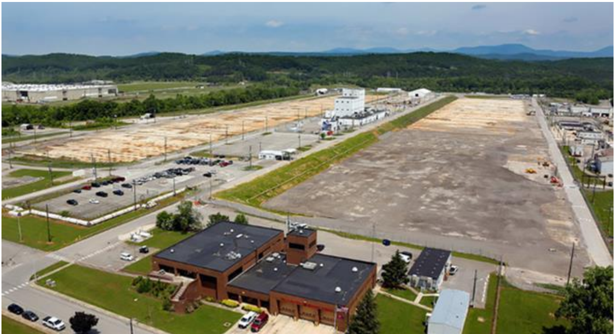
Figure 3. Building K-25 Slab, Looking North, circa 2015.
